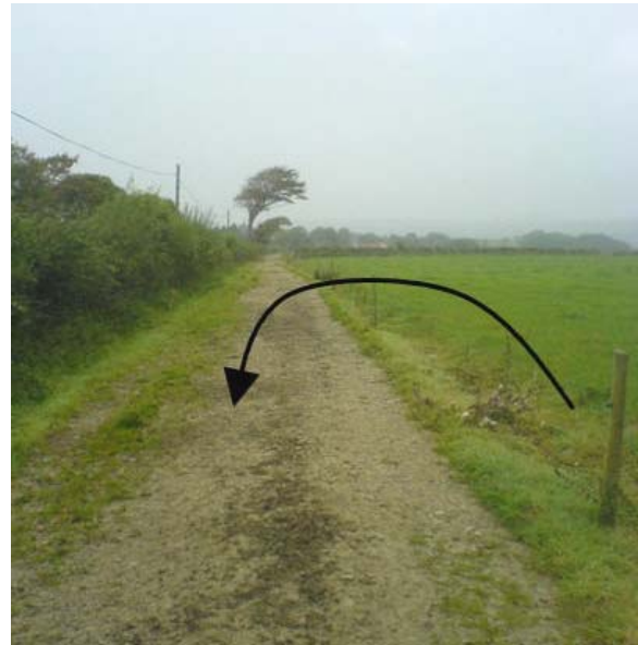
Fig 3: The 'up-and-over' involves digging up subsoil from next to the intended track, moving it over and onto the new track and back filling the topsoil
