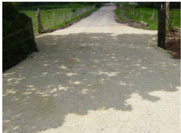
Fig 5: Oolitic limestone is a durable soft stone, that compacts well and offers excellent cow grip. Unsuitable for heavy vehicle use or high rainfall areas.
