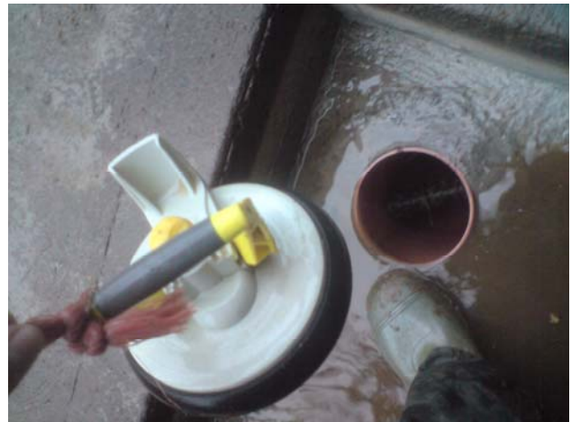
Fig 6: A 6" drain, bung and string pull.
